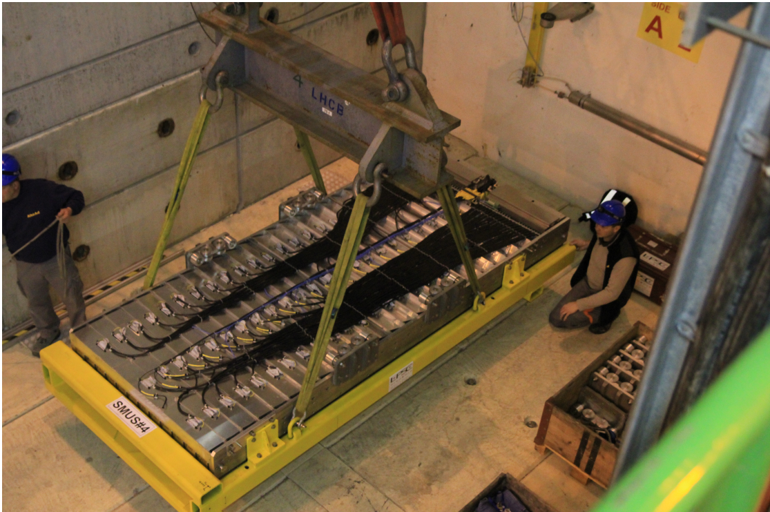
Fig. 2: View of one EMCal super-module during the installation into the ALICE detector. The cradle holds the 24 strip modules into a mechanically rigid unit. Each strip module holds 12 unit modules. On the right side the two electronics crates are visible.
